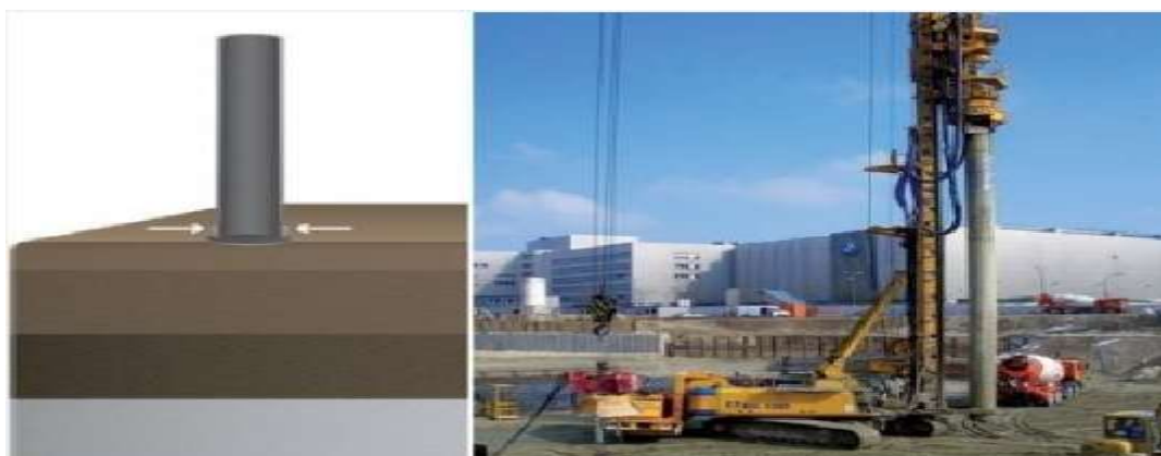
Fig.1: showing boring of cast in situ piles.
